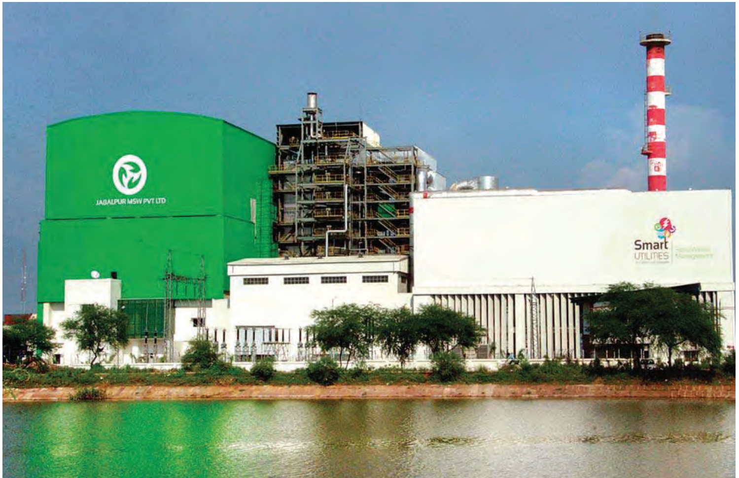
The Jabalpur waste-to-energy plant takes in unsegregated mixed feed. It can take in waste of up to 600 tonnes every day.
