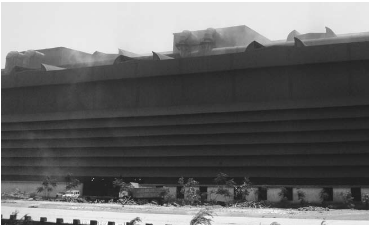
Inadequate roof dust capture system over the arc furnace unit at Bhushan Power and Steel, Sambalpur
